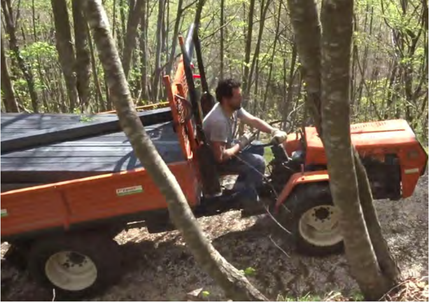
Fig.171 Screenshot showing me transporting the iron bars to the site where I have built my ark. While producing some emissions, this old tractor was indispensable. With it I was able to transport in a remote area not only the material I needed to build the ark but also the tools. In this sense the tractor did not replace my human effort but enhanced it.
